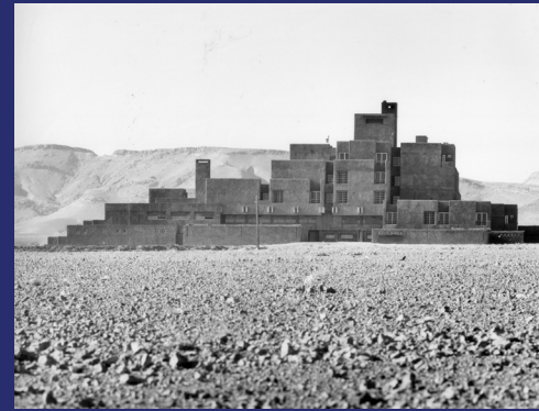
Hotel Boumalne, Studio Faraoui and De Mazières, Great South of Morocco, 1970-1971.
